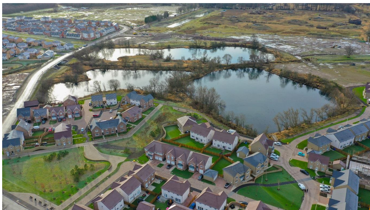
Figure 1: Aerial View of Dargavel development, January 2019 (Courtesy of Cass Associates)
